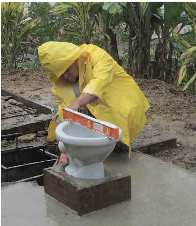
A pour-flush latrine under construction in Trojes
