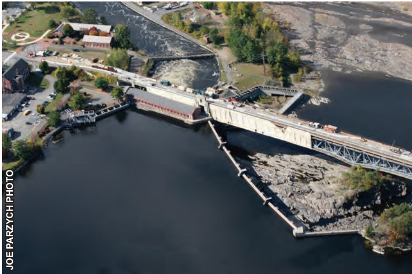
The Turners Falls dam diverts much of the river’s flow into the Power Canal.
