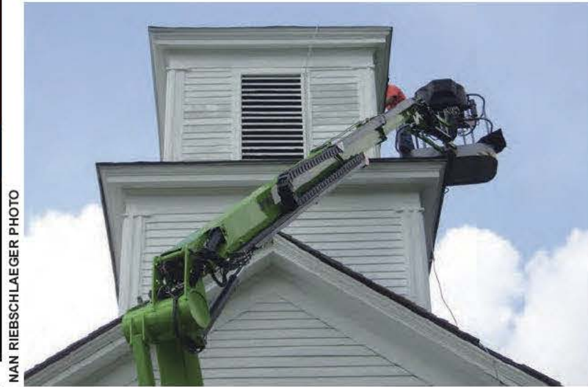
Tom Chaisson of Tri-County Construction working on the belfry of the Wendell Meetinghouse. The belfry is being repaired, painted and re-roofed. The Friends of the Wendell Meetinghouse are grateful for a generous donation that made this possible.
