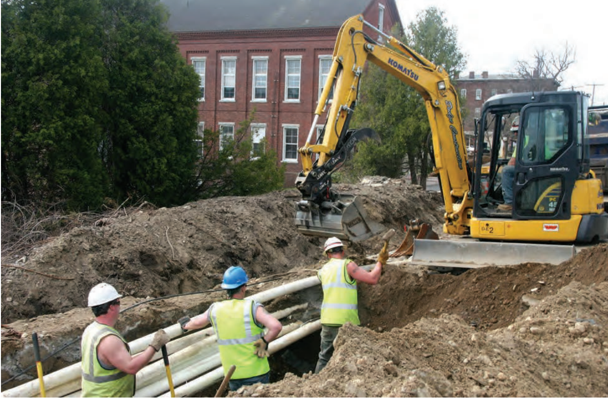
l-r Mike Biagini and Kirk Stannaway do the heavy looking on as Howard Dwerney applies gentle persuasion on some reluctant concrete surrounding cable conduits with fiber optic cables inside, while excavator operator Nate Couture waits patiently.
