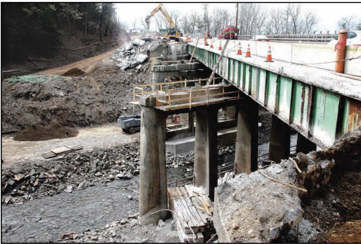
Cleaned piers were formed for the new saddles.
