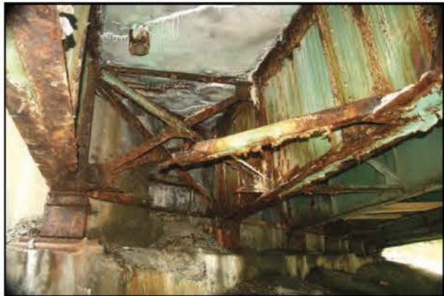
The rusted underbelly of the Factory Hollow Bridge at the start of construction.
