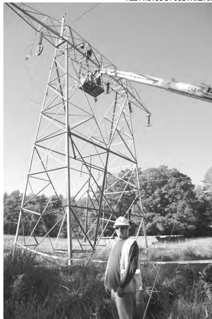
Foreman Hanes Erikson stands in front of a tower where Mario Batitis and Jameson Duncan install new insulators from a bucket.
