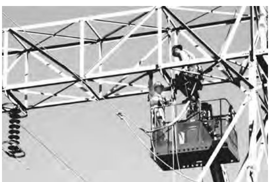
Journeymen Linemen on bi line. Mario Batitis, left, and Jameson Duncan, right, install new ceramic insulators.
