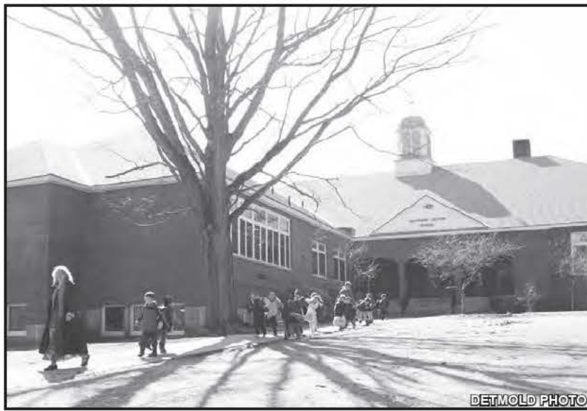
Some remember a time when the building served a purpose. This April, 2008 file photo suggests it may once have been some sort of facility for children.
