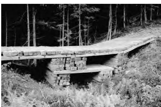
Michels Power constructed this timber mat bridge over a stream about a foot wide, as required.
