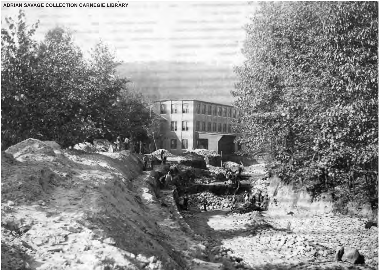
In 1903, the Millers Falls Company widened and deepened its canal substantially.
