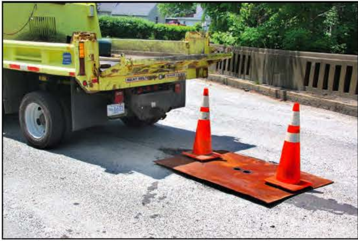
The General Pierce Bridge, connecting Montague City with Cheapside, was closed to traffic on Wednesday, indefinitely, for emergency repair. This 4' x 6' plate covers a major section of concrete that had collapsed into the Connecticut River below, leaving nothing but rebar visible. As of Wednesday afternoon, SPS New England was on the way to patch the hole, toward the end of the Greenfield-bound lane, with more fast-setting – and fast-deteriorating – concrete.
