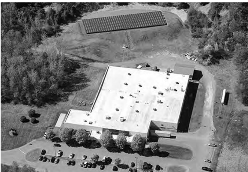
The large solar array behind the Bete Fog Nozzle plant in Greenfield has the capacity to generate 147 kW of electricity.
