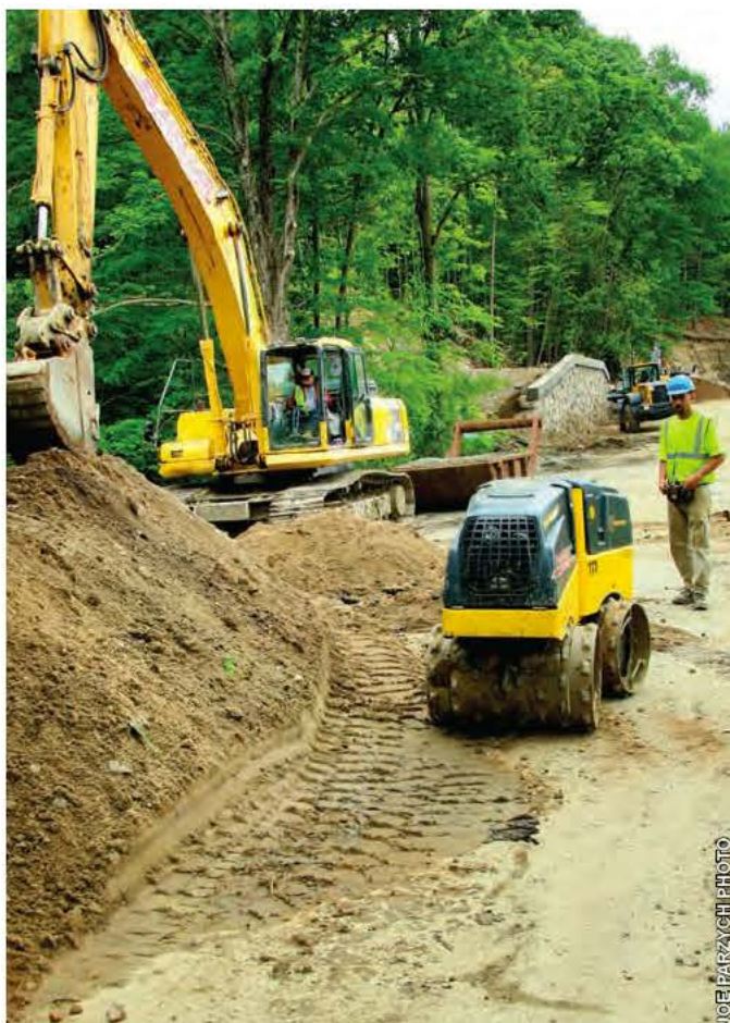
Enrique Tyson of Baltazar walking a dog – guiding a sheepsfoot vibratory roller by invisible leash remote control.
