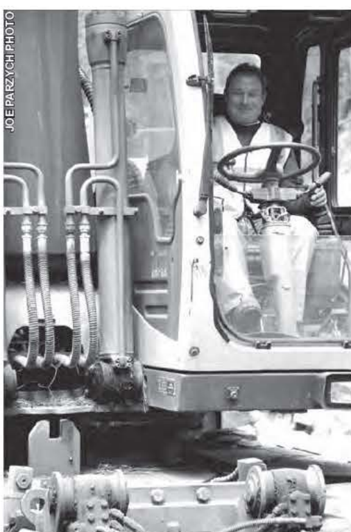
Varandas & Sons owner Gus Varandas, at the controls of his Volvo EW170 excavator, is a real hands-on CEO. The company is subcontracting under Baltazar.
