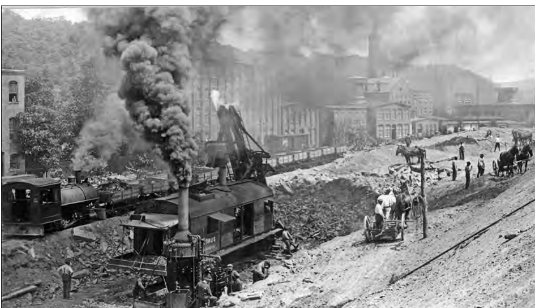
"The work on the canal is being pushed forward rapidly and much progress is being made..." The photo at left shows the work to enlarge the power canal, in order to extend it to Cabot Station. On September 10, 1915 the west bank collapsed due to a lining failure. Photo used by permission of Peter S. Miller. At right, the canal on July 1, 2015; Mike Jackson photo.
