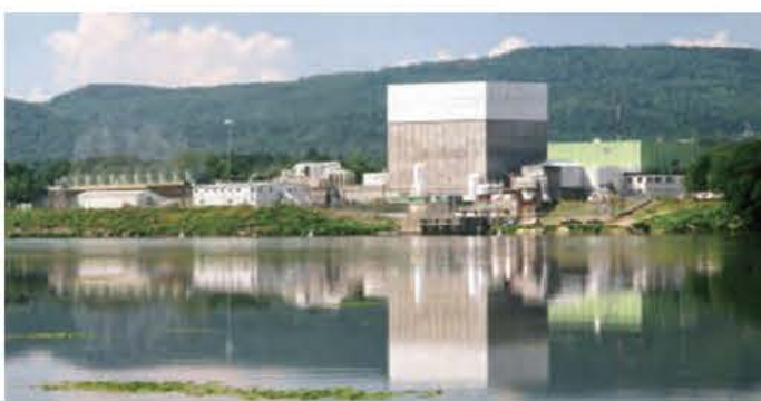
In August, Entergy announced it would stop producing power at the Vernon plant in December 2014.
