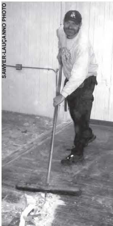
Co-owner Chris Sexton cleaned up the new storefront on Monday.
