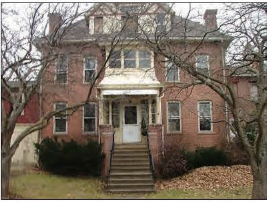
St. Anne's Rectory, on J Street, has no internal plumbing, HVAC, or elevator.
