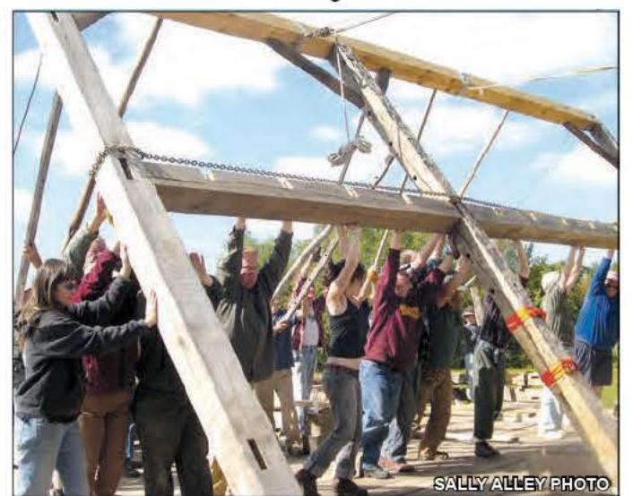
Since this 2008 barn raising, the von Ransons have sought approval to live without electricity or standard plumbing in their apartment.
