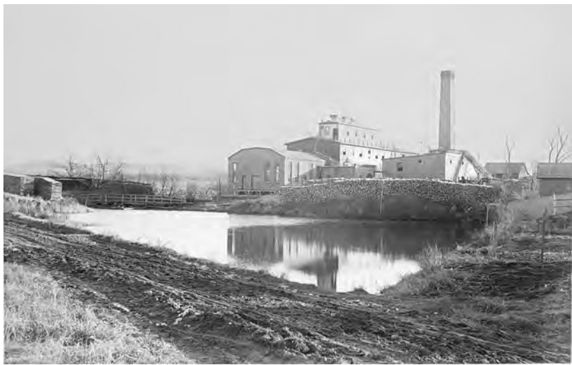
The New England Fibre Co. pulp mill was built behind Fort Hill in 1886, along with a pond created by damming up Heal-All Brook. The pond water was pumped into the mill, heated, and used for steam power. Note the piles of firewood used for fuel.
