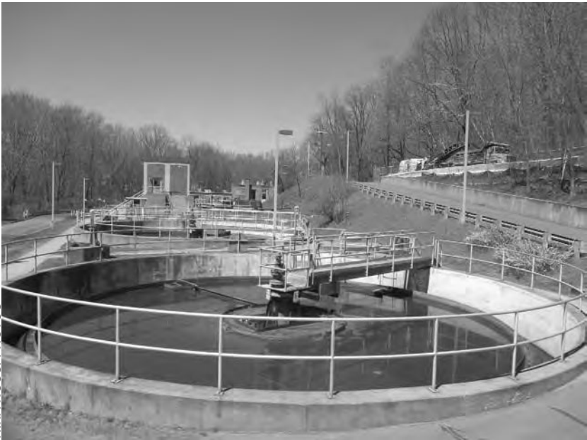
A secondary clarification tank at the Greenfield Road facility.
