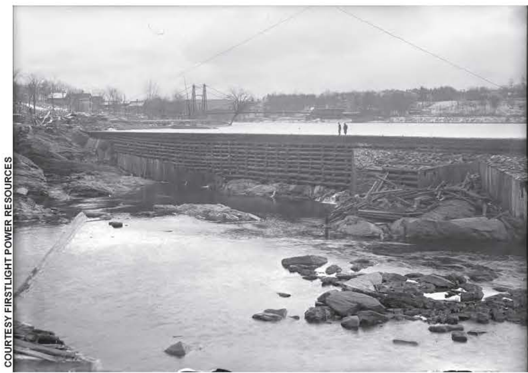
This 1915 photo was taken from the top of the newly constructed dam, looking upstream at the older stone-filled crib dam built in 1866. The old suspension bridge can also be seen in the distance.
