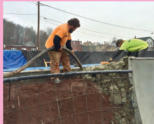
Grindline supervisor Eddie Lawrence pours concrete into the transition between the park’s full bowl and the bowled portion of its street section in December.
