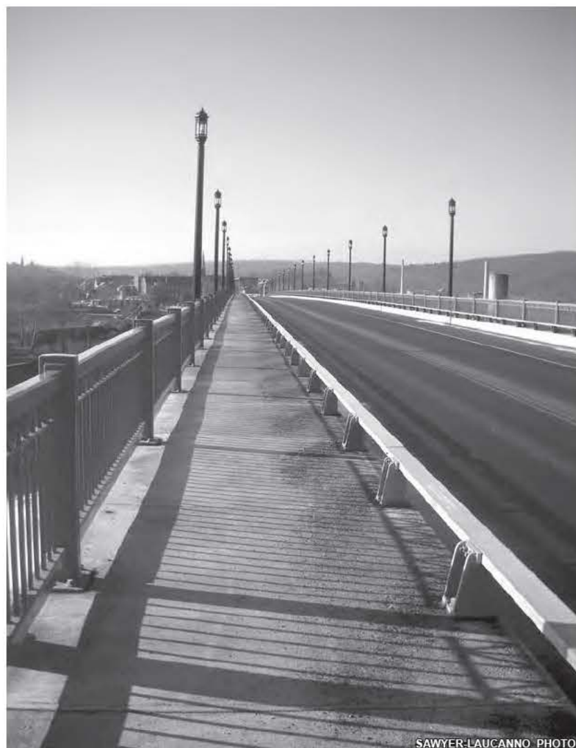
Who will plow it? The Turners Falls-Gill bridge's sidewalk awaits a decision.
