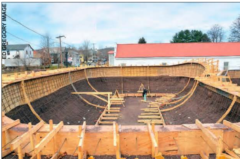
Ed Gregory shared this picture of progress on Unity Skatepark. Curved rebar holds the shape of the park's main bowl.
