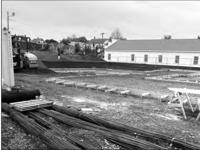
As of this Wednesday, the fill was graded, and wood framing was being constructed to pour the concrete bowl planned for the park’s northern end.
