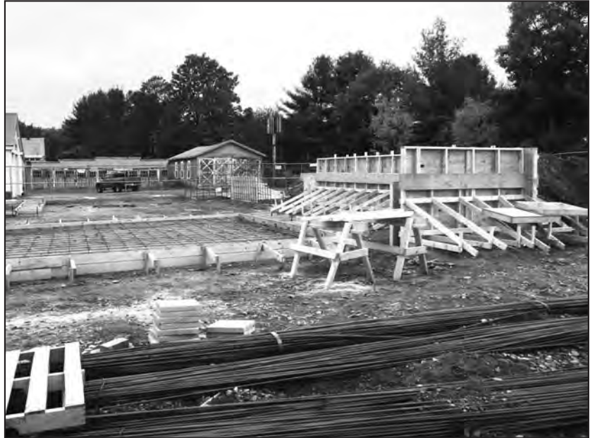
As of this Wednesday, the fill was graded, and wood framing was being constructed to pour the concrete bowl planned for the park’s northern end.
